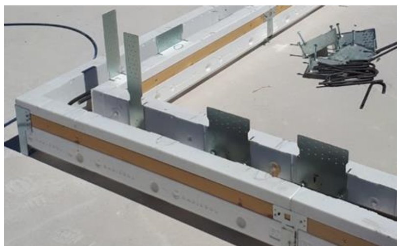
Installation of SLP20 and HD50 structural brackets
