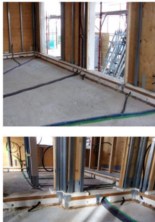
Pipes laying with RADICSOL
