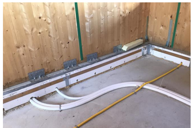
Horizontal pipes passages
