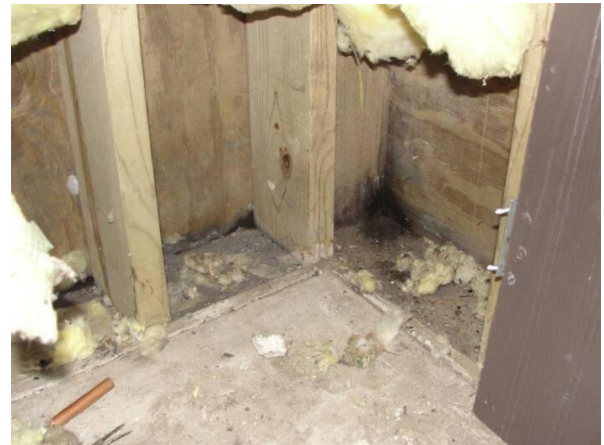
INTERSTITIAL CONDENSATION DAMAGE
