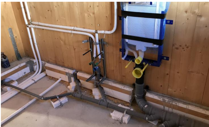
Wall pipes passages
