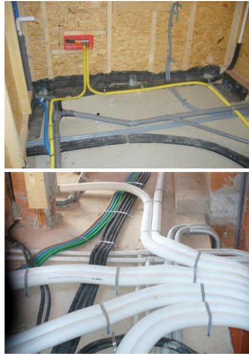
Pipes laying with traditional curb or without curb
